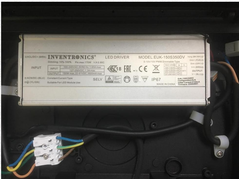
Figure 6 (Label of the LED driver)
